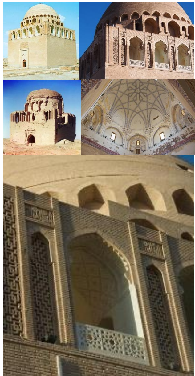
Figure 5. Mausoleum of Sultan Sanjar reflects innovative technology, integrating Hazārḃāf brickwork, tile revetment, and painting into a unified structure with symbolic depth. (Photos: authors' archive).
