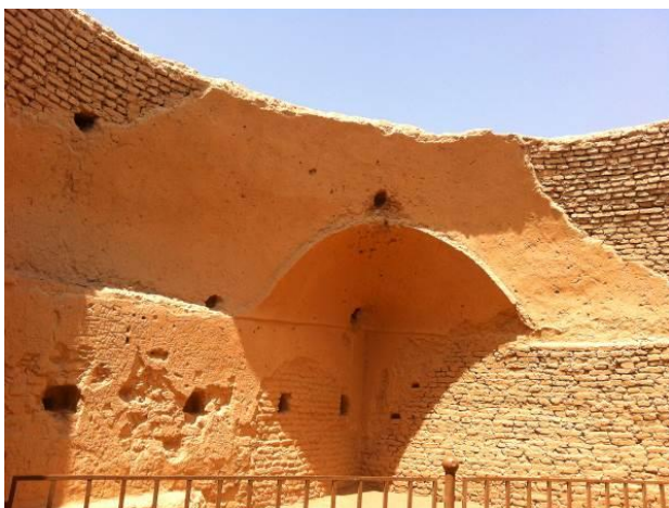
Figure 10. Adobe Brick Construction
