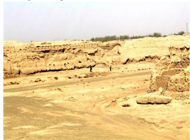
Figure 3. Outer City Wall
