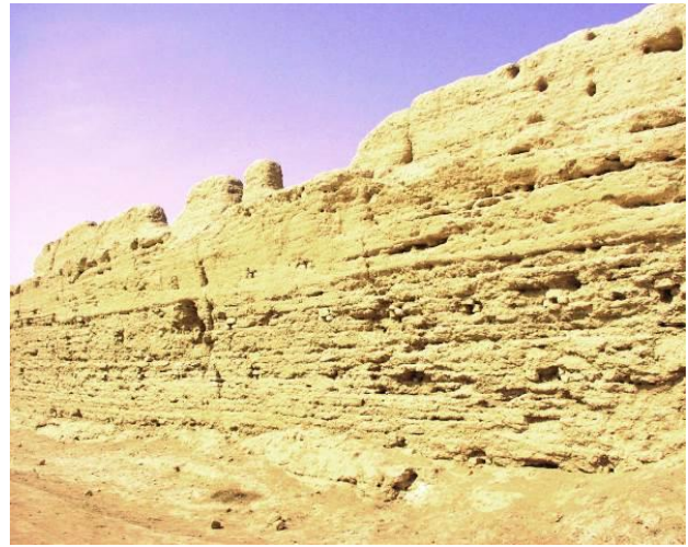
Figure 9. Rammed Earth Wall of the Ancient City of Gaochang
