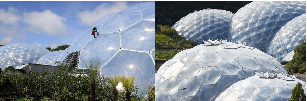
Figure 3. The Eden Project in the UK uses ETFE foil cushions allowing high light transmittance and insulation (Archdaily, 2024).
