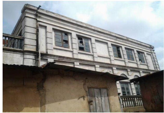
Figure 4: Side view of the building
