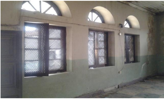
Figure 11: Glass windows with wooden finished blind
