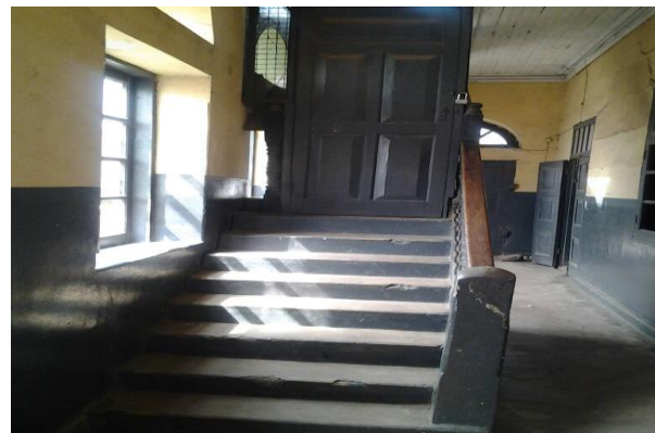
Figure 16: Wooden door used as security to upper start of the staircase
