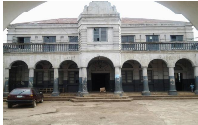
Figure 8: Approach view of the main building
