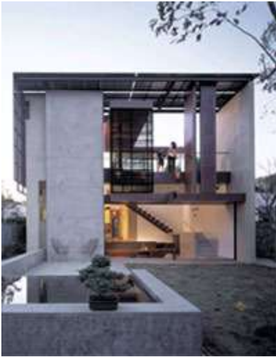
Fig 5: Solar Umbrella House Source: Courtesy of Brooks and Scarpa Architects
