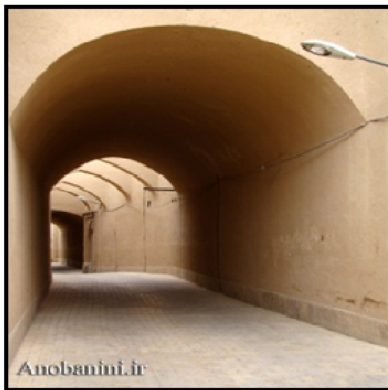
Figure 2: Covered Passage - The Old context of Yazd
