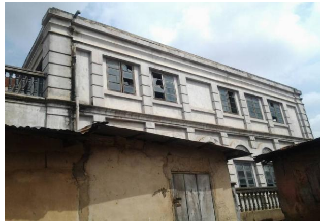
Figure 4: Side view of the building
