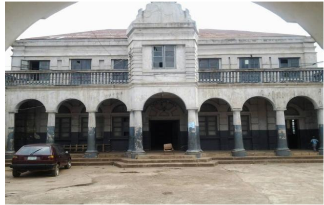
Figure 8: Approach view of the main building
