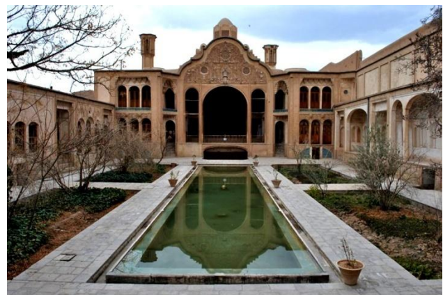
Figure 2. the main yard, the connection of human and nature, Borujerdis' house, Kashan
