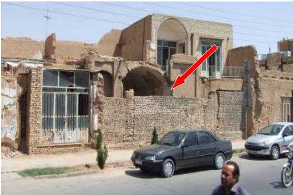
Fig 12: a half destroyed building on the edge of Basij Boulevard
