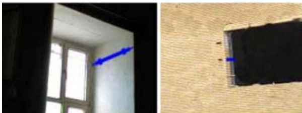
Fig 5. reducing the thickness of the walls in the new buildings
